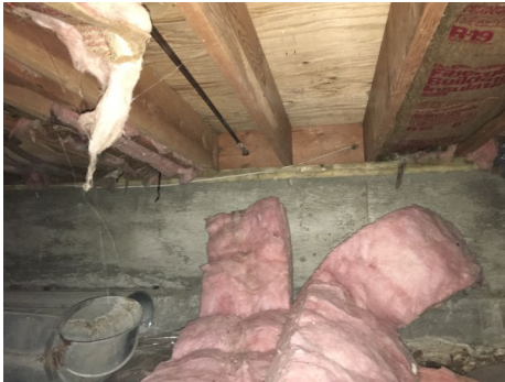
Mold under improperly installed insulation
