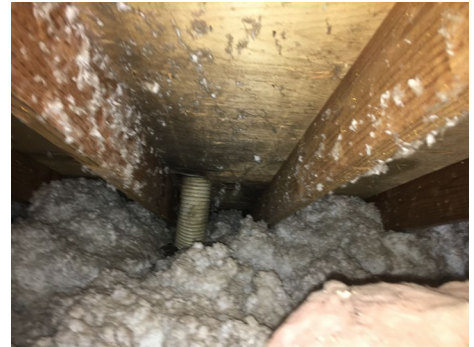
Mold in attic where duct is not properly vented.
