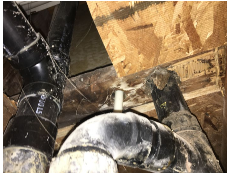
Mold under previous bath tub leak
