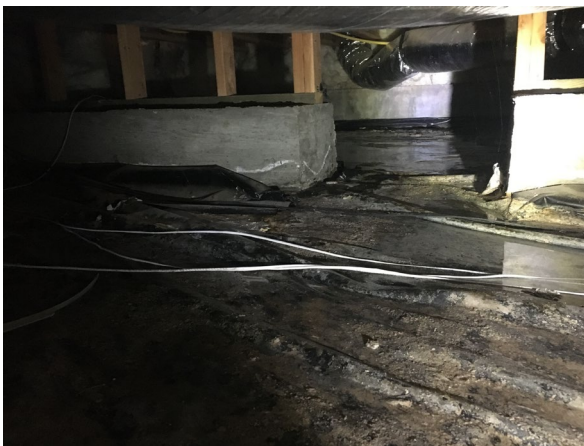
Standing water on top of the vapor barrier
