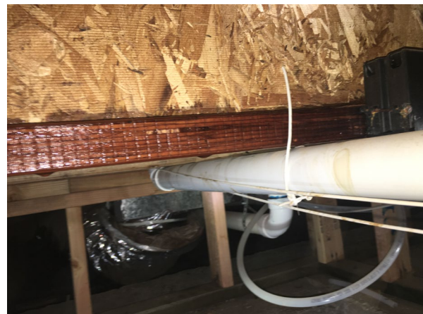
Active leak from refrigerator
