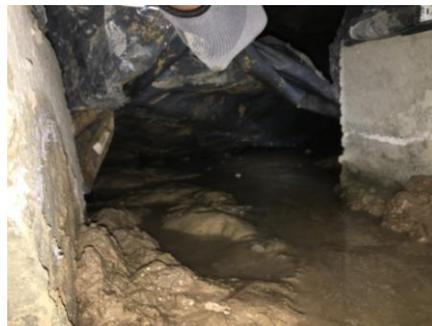
**standing water/mineral line indicates water level from repeated intrusion**
