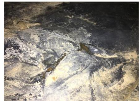
**Water damaged vapor barrier**
