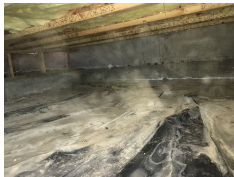
mineral line and damaged vapor barrier
