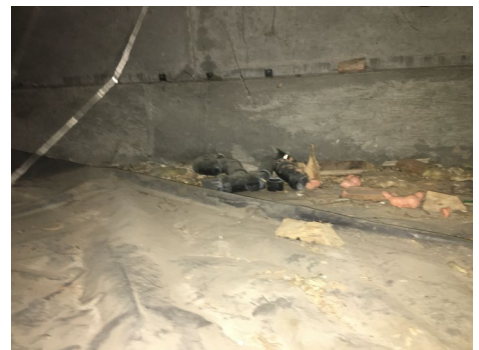
debris and damaged vapor barrier
