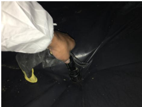
standing water under vapor barrier
