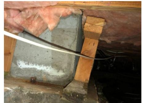
water damaged pony wall- side view- tilted
