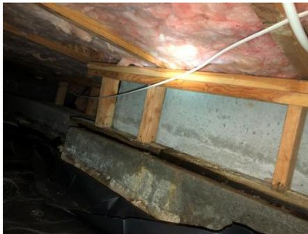
water damaged pony wall-front view
