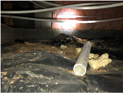
Debris under remodeled bathroom
