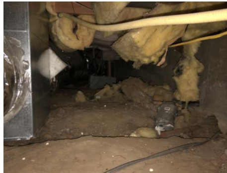
misc. debris and missing vapor barrier
