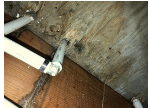
mold on floor decking
