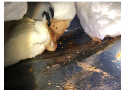
Wet insulation at the bottom
