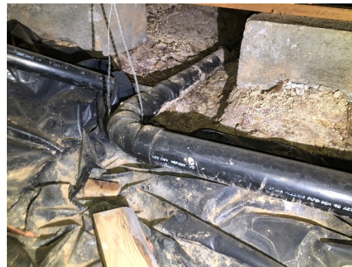
Mineral build up from repeated intrusion/drying
