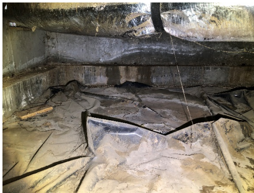
Water lines at cold joint from repeat intrusion
