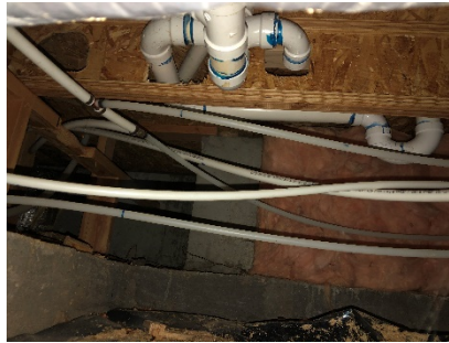
Notched for plumbing
