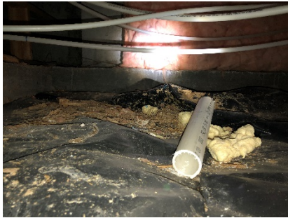
Debris under remodeled bathroom
