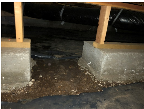
Water intrusion/Poor vapor barrier
