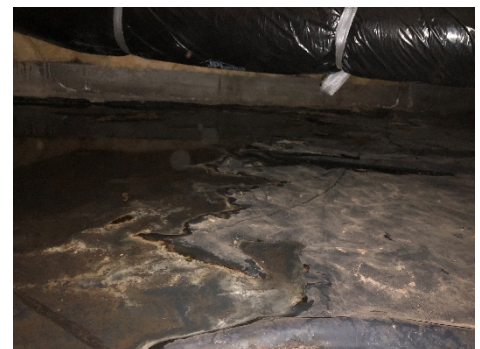
Standing water/Poor vapor barrier
