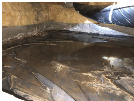
Standing water/Poor vapor barrier
